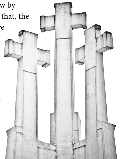
Crosses on Three Crosses Hill
